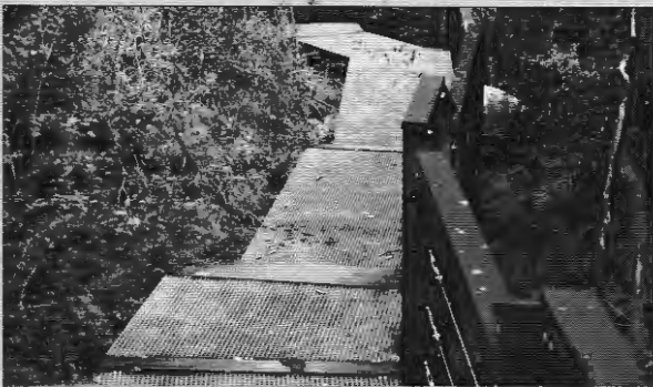
2010 track construction — non-slip grillage, timber-framed handrails, wire stringers with stainless steel turnbuckle tensioners. Captain Abbott would have loved it.
